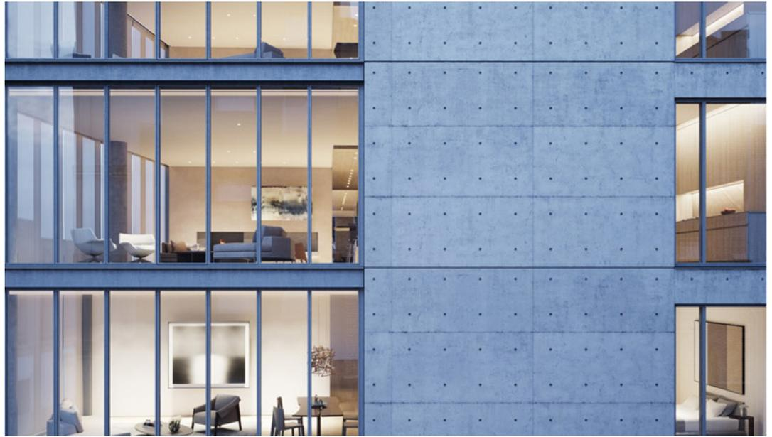
In between the expanses of concrete, floor-to-ceiling glazing is underlined by steel I-beams that bring to mind Mies van der Rohe's own brand of structural expression. A series of columns (concrete, naturally) provide structural support for the floor plates, allowing for super-slim mullions and slender corner details in the vein of Place 57, designed by luxury condo connoisseur Ismael Leyva.
