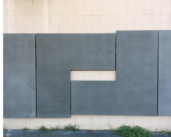
Long pieces of L-shaped concrete cladding will form the exterior of 30 Warren.
